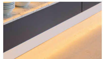
LED lighting plinth
